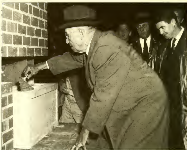
Dr. Turner lays mortar on the cornerstone, October 10, 1951. Standing beside Dr. Bowen is architect A. C. Woodroof.
